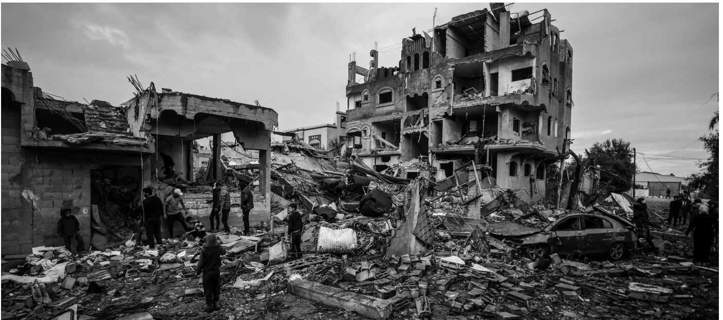
Huge destruction was left in the Maghazi camp in the central Gaza Strip following an Israeli massacre that killed 70 people, Photo: Ali Jadallah, Anadolu Agency - December 24, 2023
