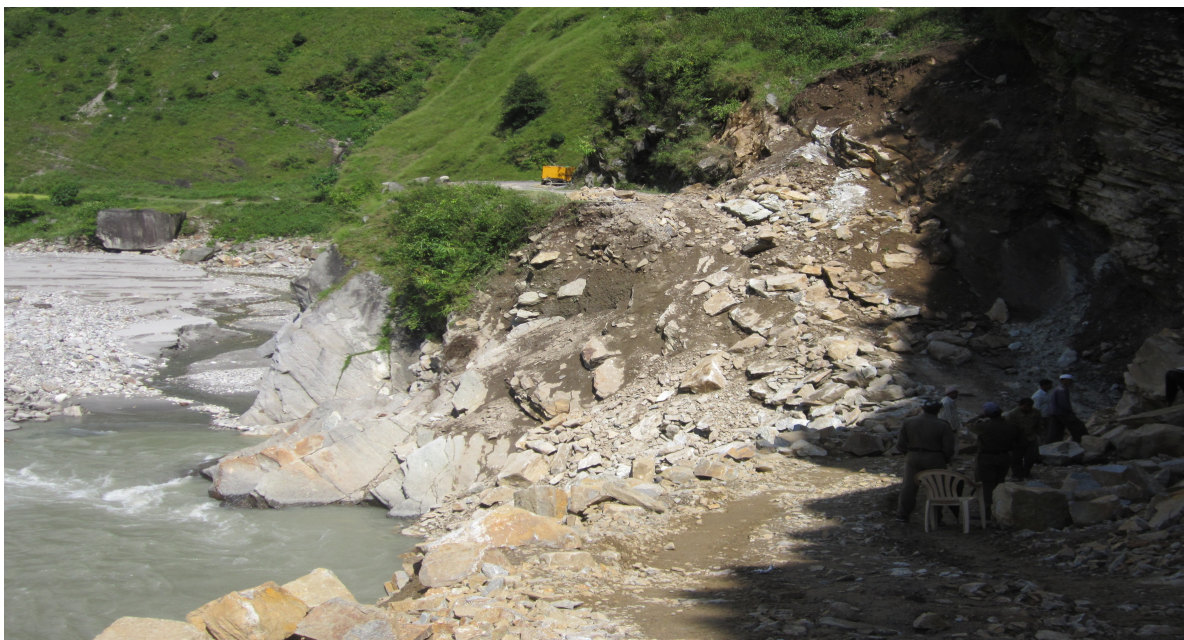
Massive destruction of roads connecting far off villages. The relief and rehabilitation measures have still not reached to places where it was most required.
